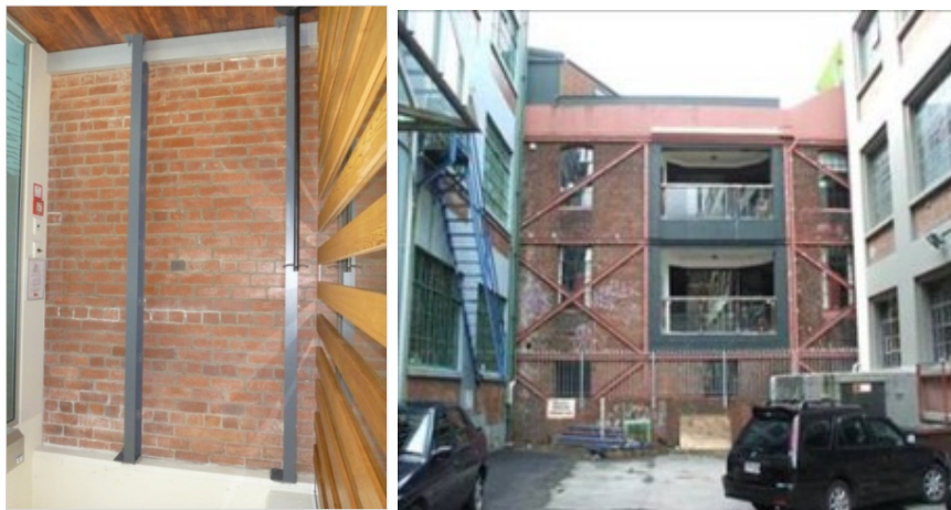
Figure 7 Anchoring steel posts or frames to increase in-plane and out-of-plane flexural capacity (NZSEE et al., n.d.-c)
