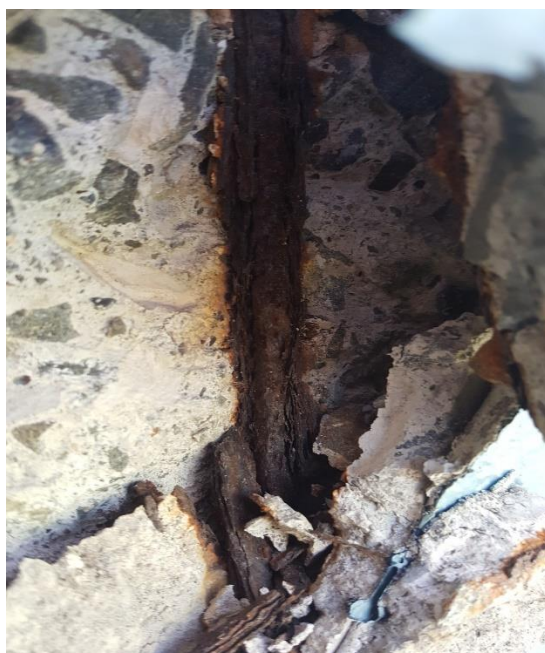
Corroded Reinforcement
